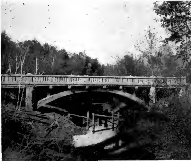
The White Mud River arch bridge is the first of its kind in Manitoba and a type well suited to the needs of the province
